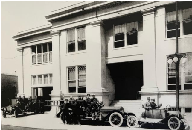
Old City Hall/fire station number one (Circa mid 1920s)
