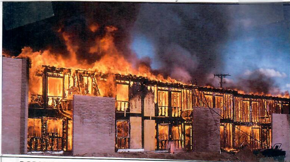
DORADO APARTMENTS FIRE, EAST CENTRAL AVE. NE (1973) (Photo By: Dave Windle, 1973)
