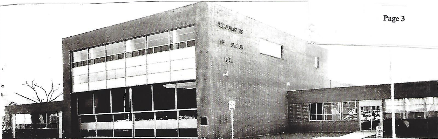
ALBUQUERQUE FIRE STATION # ONE 8 TH STREET & SILVER AVENUE S.W. CIRCA (1957)
